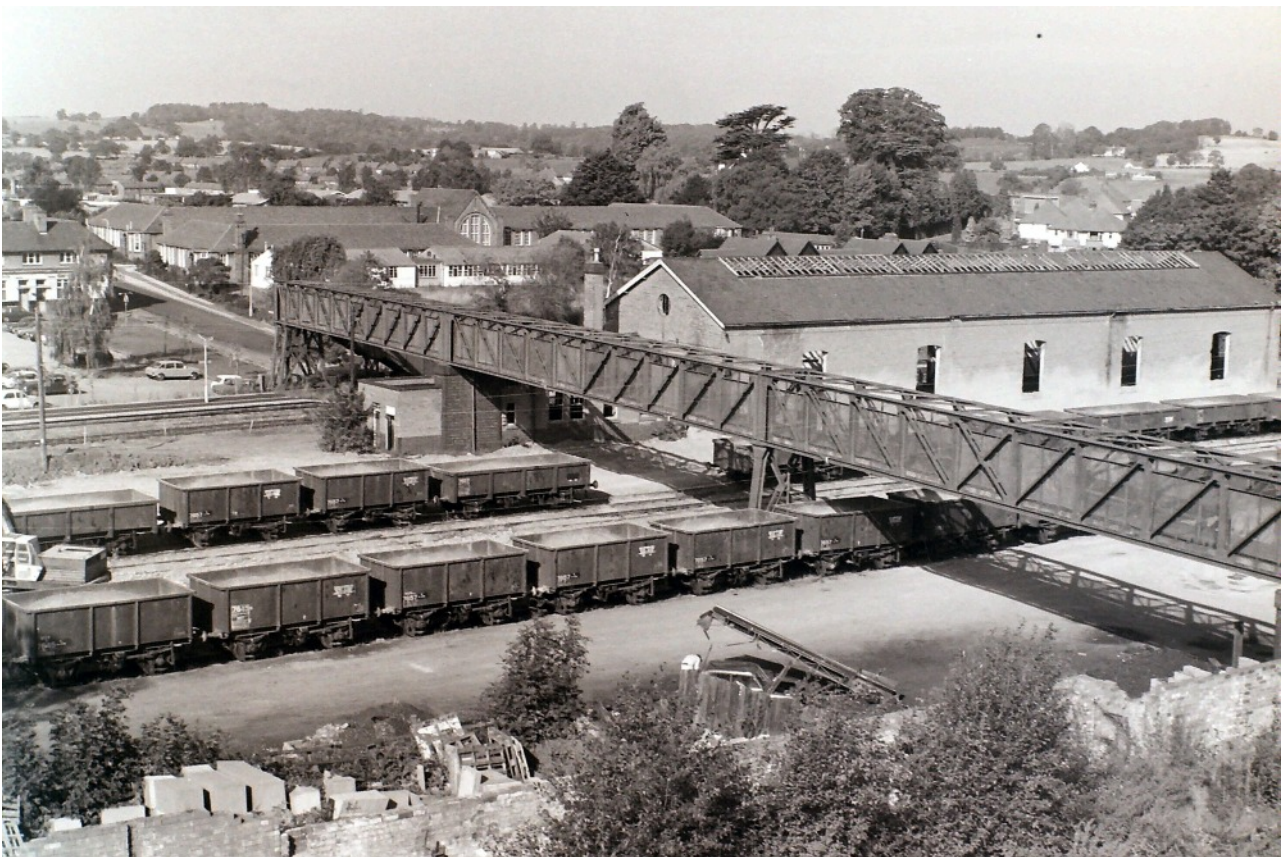
Railway Goods Yard - Railway Trucks loaded with Ballast for New Town construction work.
