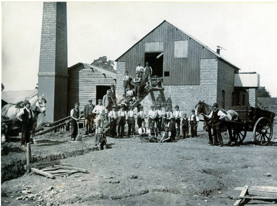
Ferny Hill Brickworks - A group of workers outside the Ferny Hill Brick works. It is believed these are construction workers building or extending the facilities rather than brick makers.
