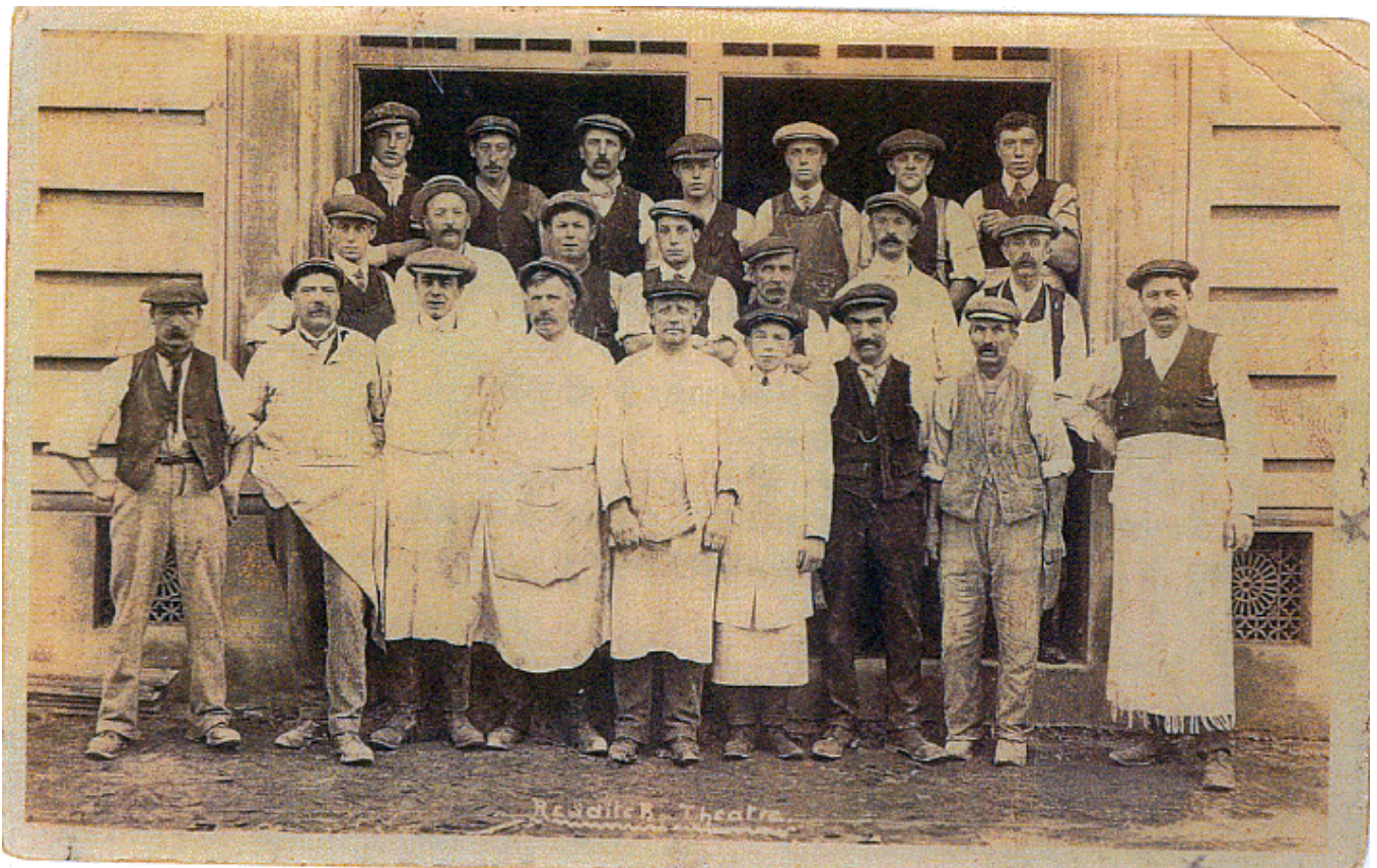
The Palace Theatre - 1913 The New Theatre and the workers who built it.
