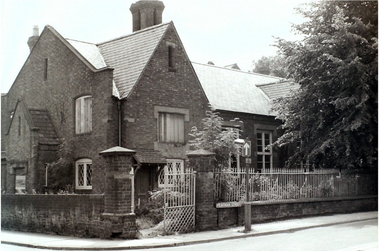
Peakman Street - Clearly Peakman Street and St. Stephen School.
