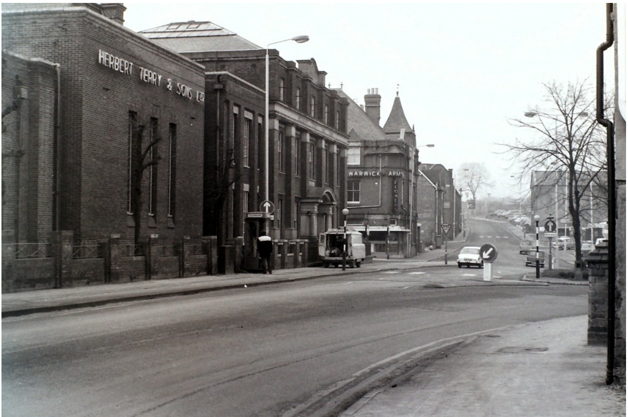
Ipsley Street - Millsborough House looking West.
