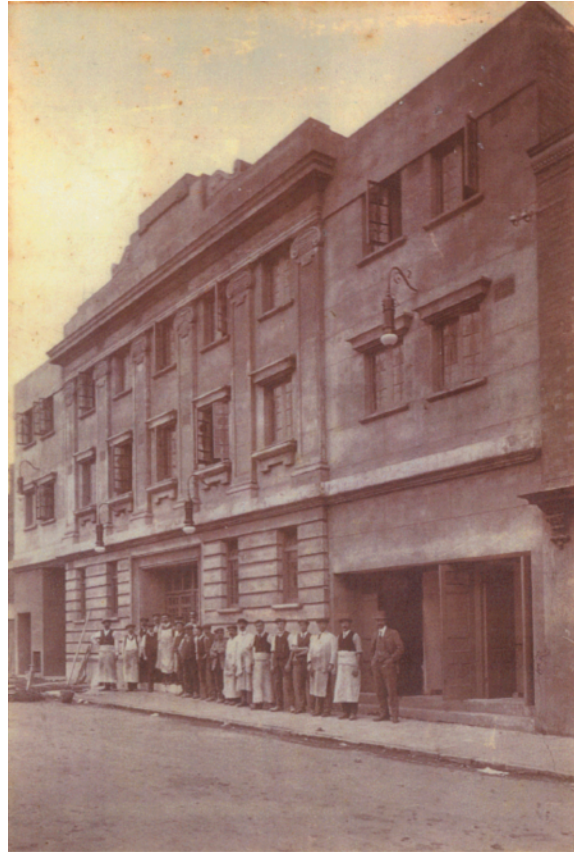
The Palace Theatre - 1913 The New Theatre and the workers who built it.
