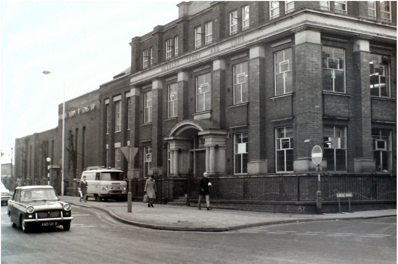
Ipsley Street - Millsborough House looking East.
